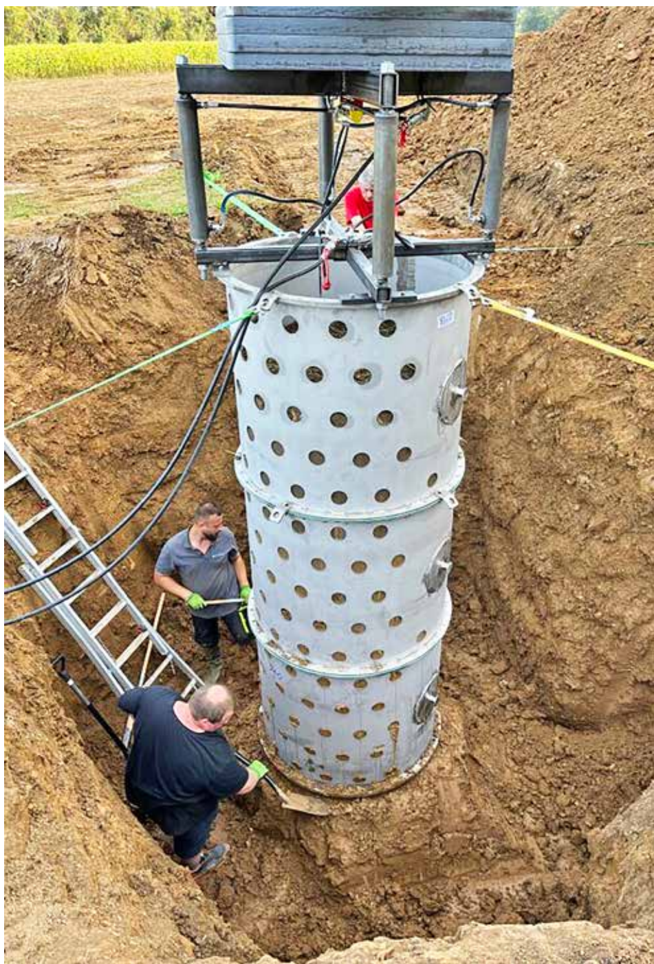
The University of Idaho's $25 million Deep Soil Ecotron will include 24 of these "eco-units" that will hold eight tons of soil each and be used to conduct research on deep soil properties.
