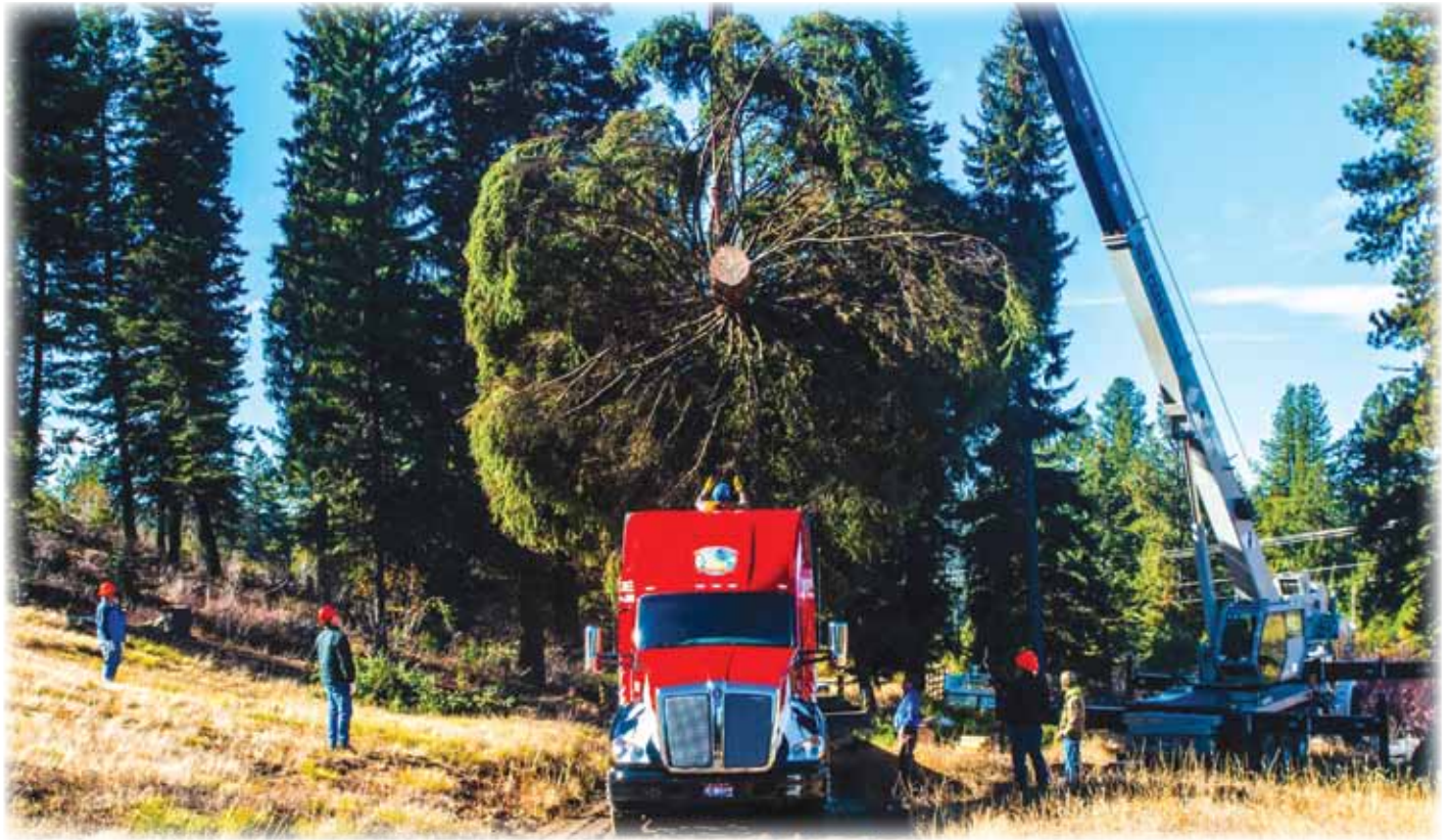
A crane was used to place the tree in a specially made cradle on a flatbed trailer.
