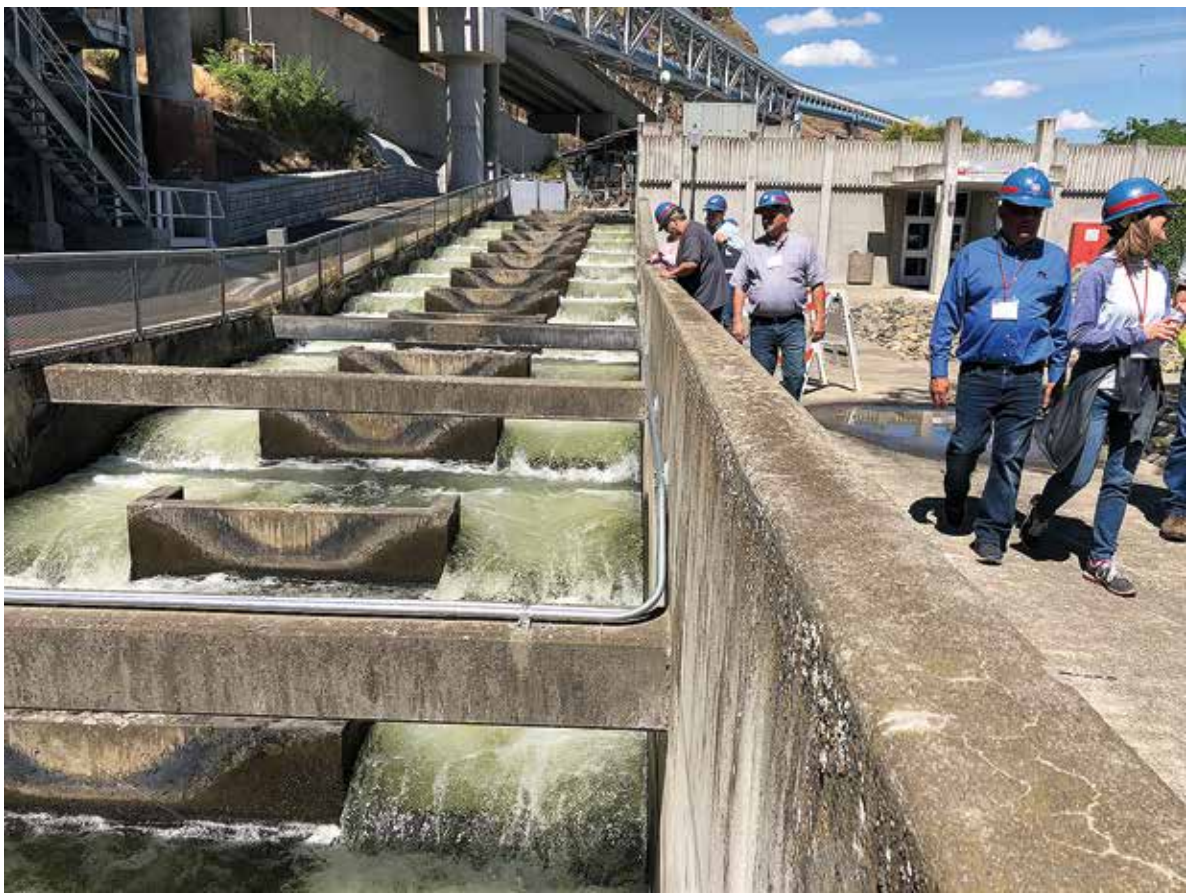
During a tour of Lower Granite Dam on the Snake River June 16, state, regional and national agriculture industry leaders viewed a fish ladder, which helps endangered salmon make their trek through the Columbia-Snake River system.
