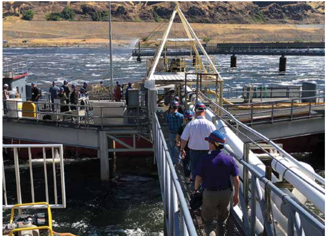
During a tour of Lower Granite Dam on the Snake River June 16, state, regional and national agriculture industry leaders tour a barge that moves endangered salmon up and down the Columbia-Snake River system. a fish biologist discusses some of the efforts being undertaken to help endangered salmon survive their trek up and down the river system.
