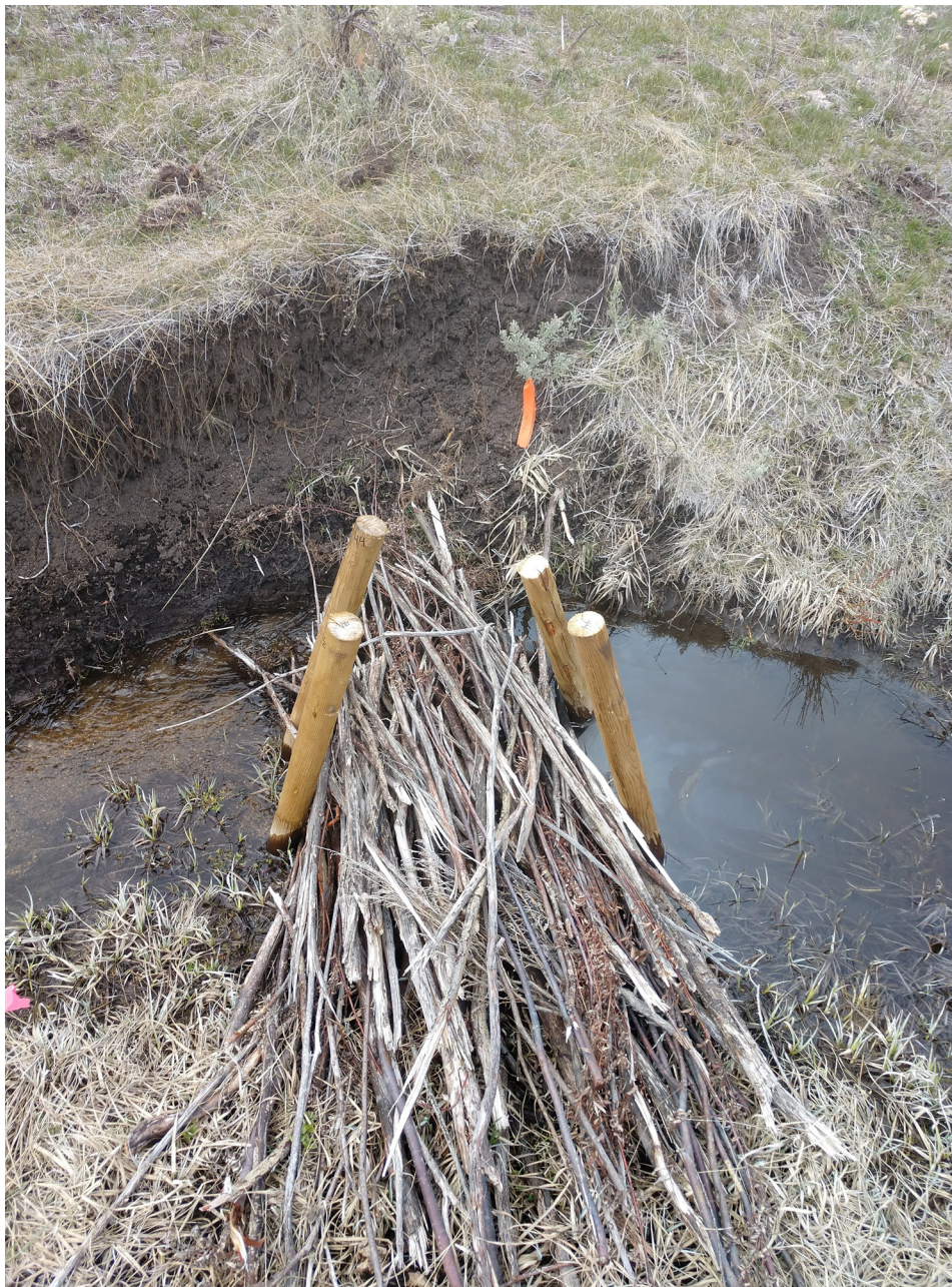
A beaver dam analog at University of Idaho's Rinker Rock Creek Ranch.
