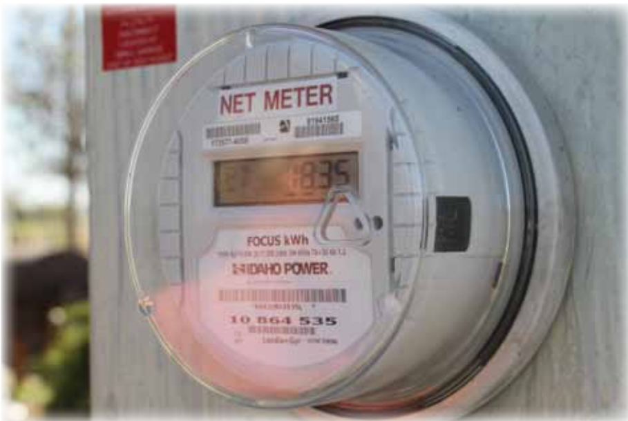
A net metering device detects when the on-site alternative energy production exceeds a home's grid power usage. The meter then spins backwards, earning the homeowner power credit.
