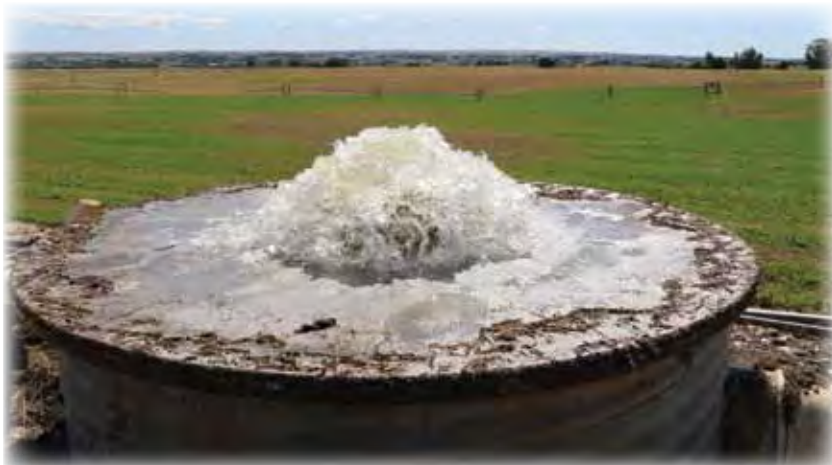
A bubbler boils up irrigation water on the Emmett bench in Gem County. The water boils up and drops through a screen to remove debris from the water before feeding into ditches and onto crops.
