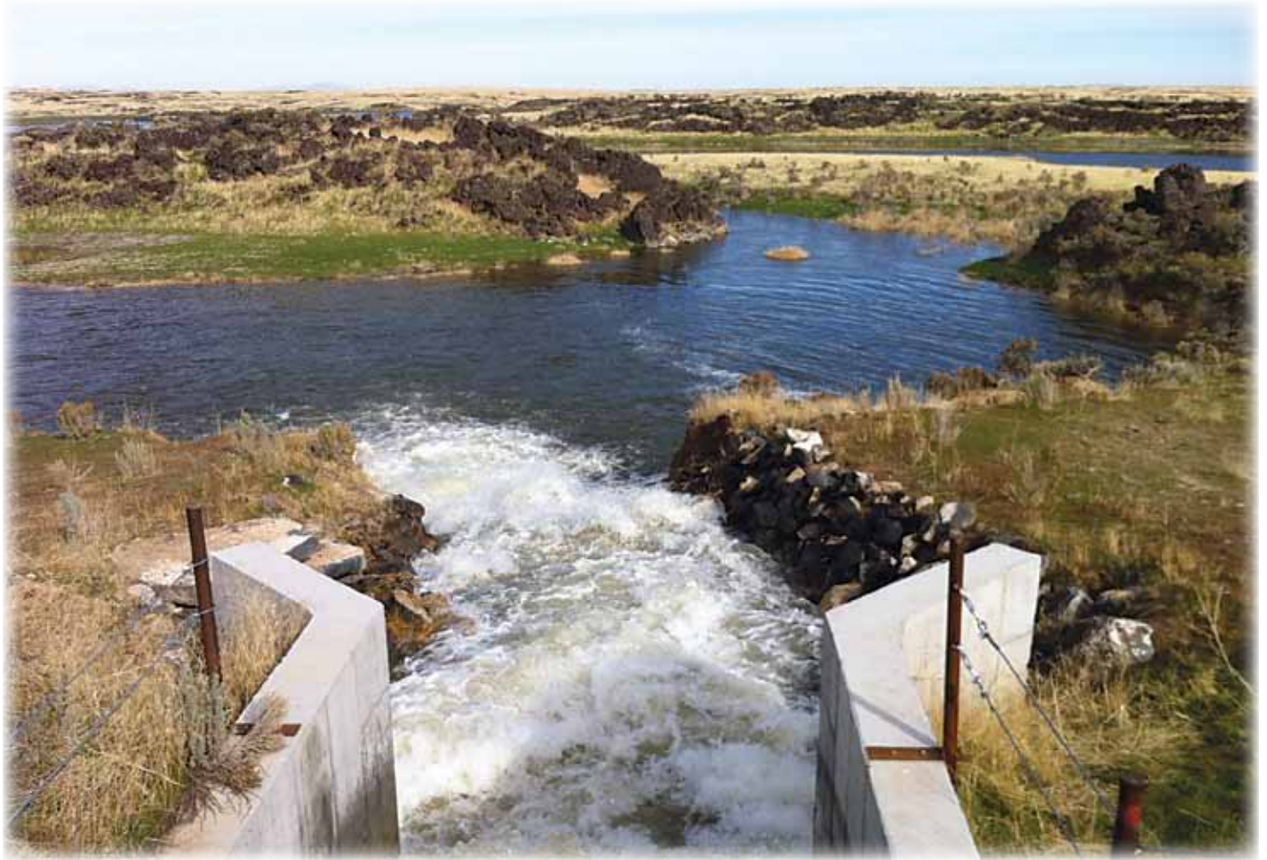
Water flows into Milepost 31 Recharge Site off the Milner-Gooding Canal. Photos courtesy of Idaho Department of Water Resources
